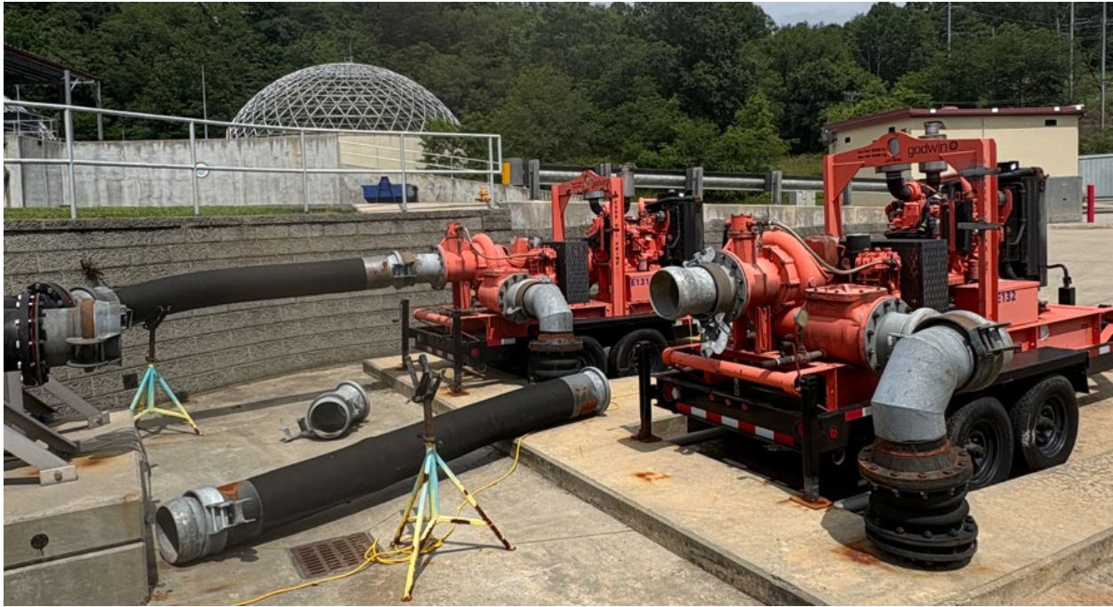
Picture 3 - WRF Bypass Setup
