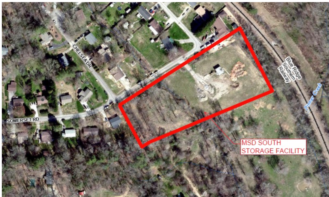
Picture 1 - MSD South Storage Facility
